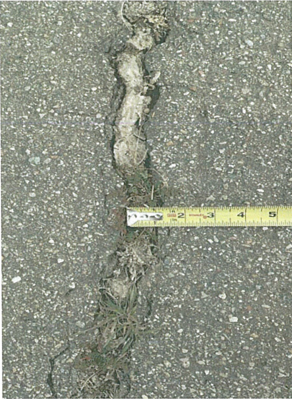
Photo 3: Width of asphaltic concrete surface crack at station 118+00.
