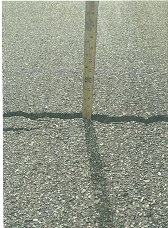
Photo 4: Depth of asphaltic concrete surface crack at 138+00. (Note: inverted 18-inch tape measure used in photo.)
