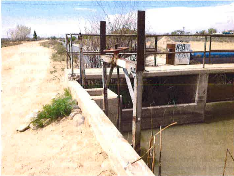
Figure 2. Helium Siphon Turnout to be Replaced
