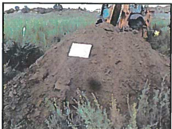
Test Pit TP-23
