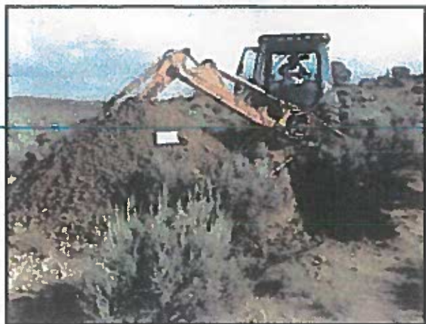
Test Pit TP-13
