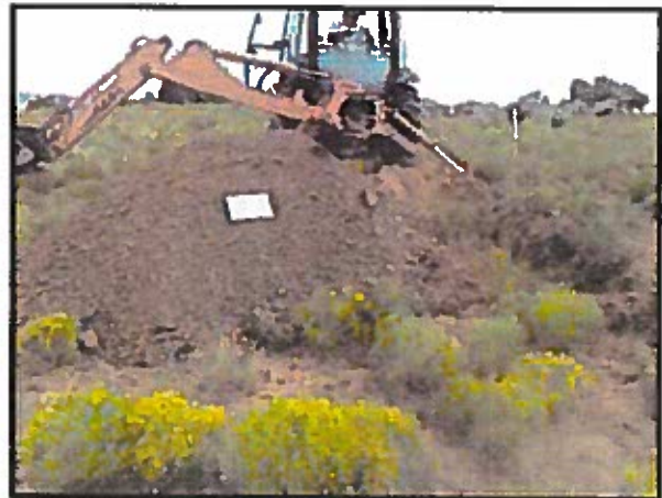
Test Pit TP-21
