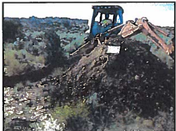
Test Pit TP-12
