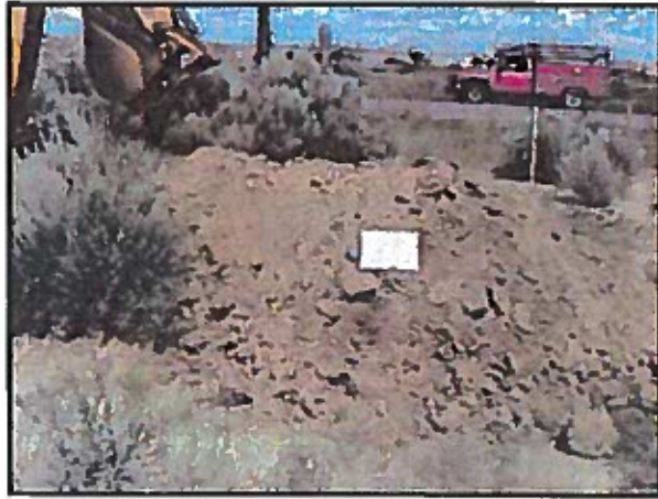
Test Pit TP-20
