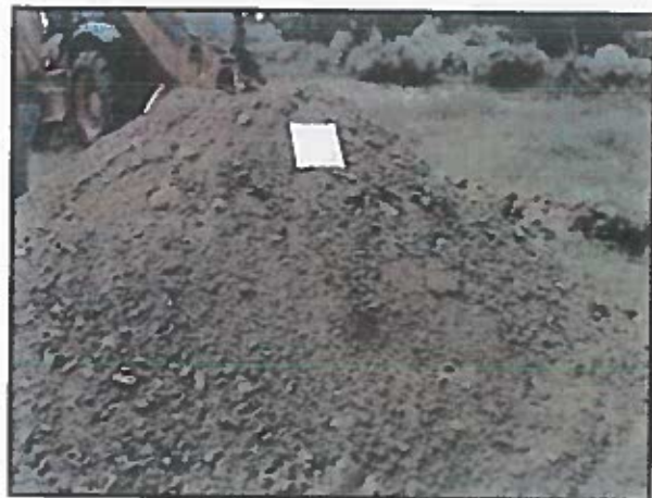
Test Pit TP-3
