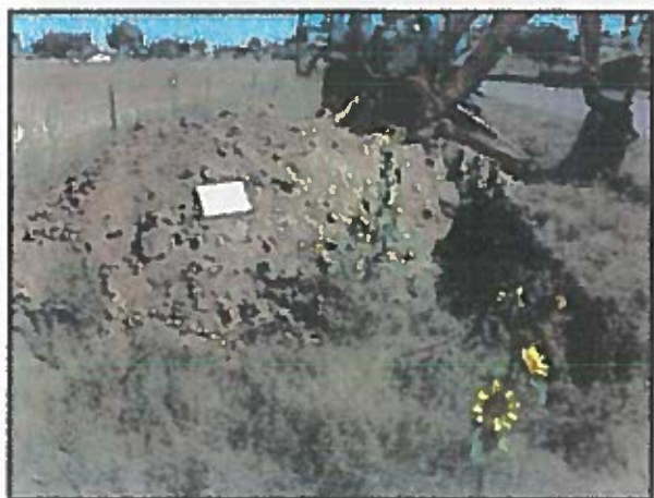
Test Pit TP-16
