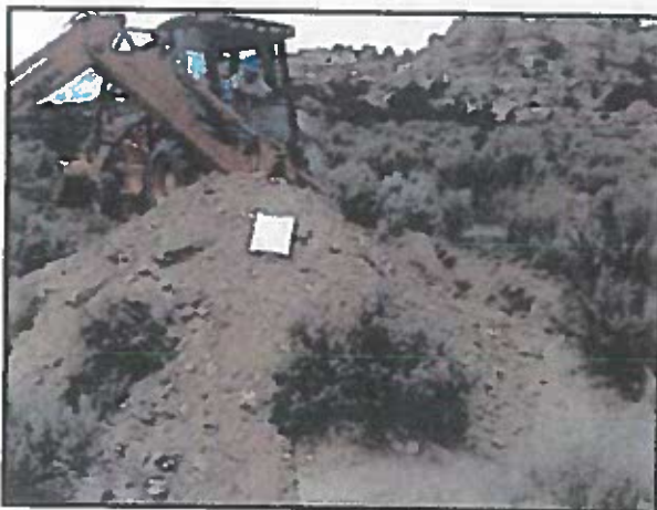
Test Pit TP-2
