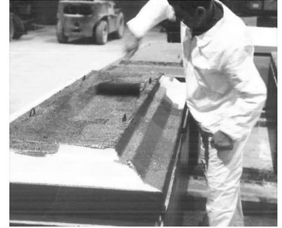
Water Based Damp Proof Coating for Concrete
