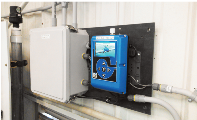
Typical installation with mounting bracket
