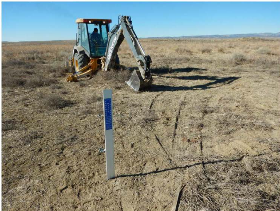
Test pit excavation along the line pipe alignment of Reach 10 near Pumping Plant 7.
