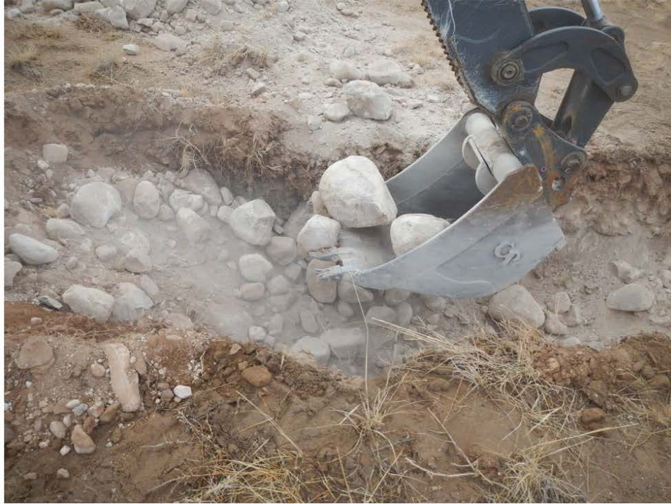
Excavation of cobbles and boulders in test pit TPSTR7-16-5. Image for reference only.
