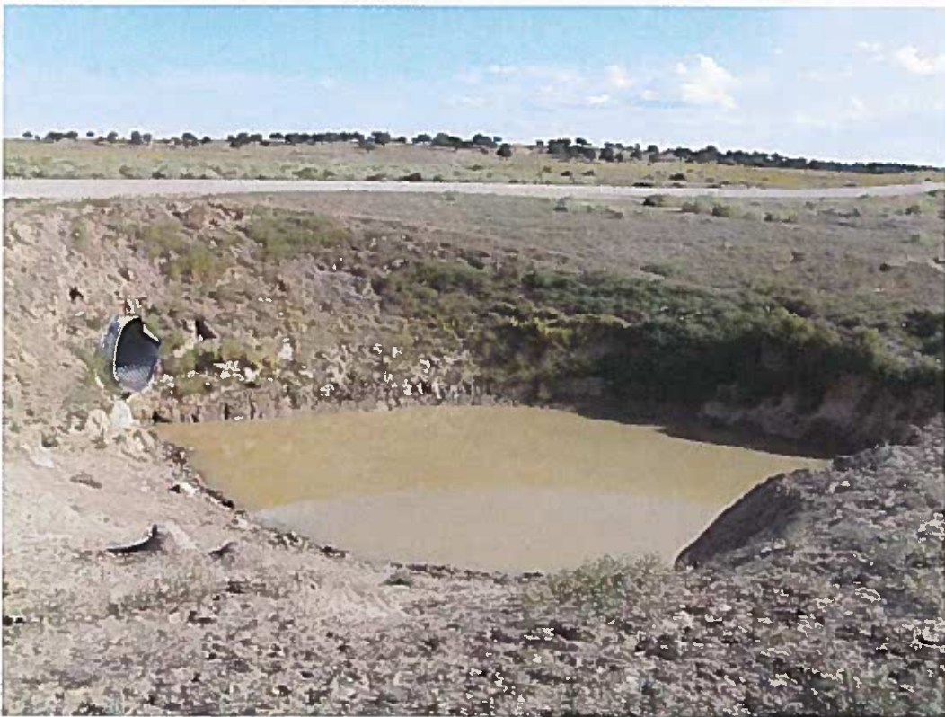
Photos 3 and 4: Drainage Culvert Located approximately 65 m (213 ft) south of station 3+965 (note standing water)
