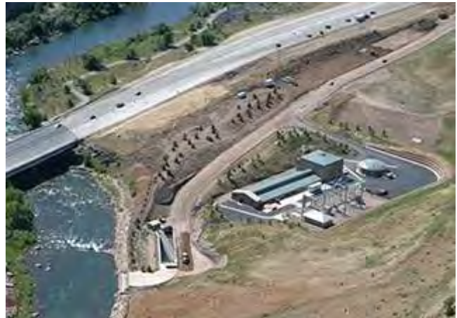
Aerial view of the Durango Pumping Plant
