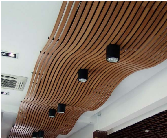
Figure 21 – Curved Wood Ceiling
