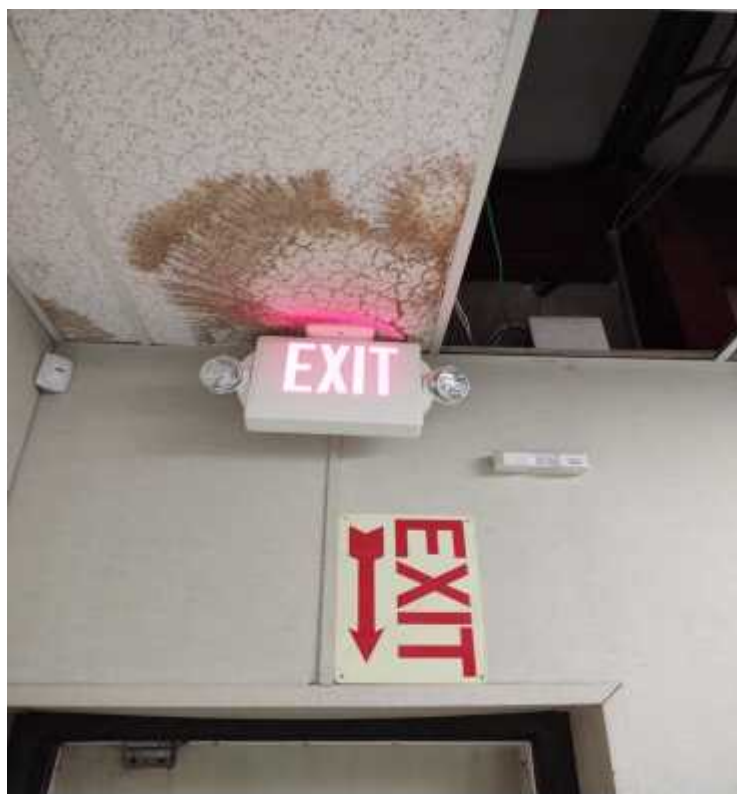
Exit Door on West side of building
