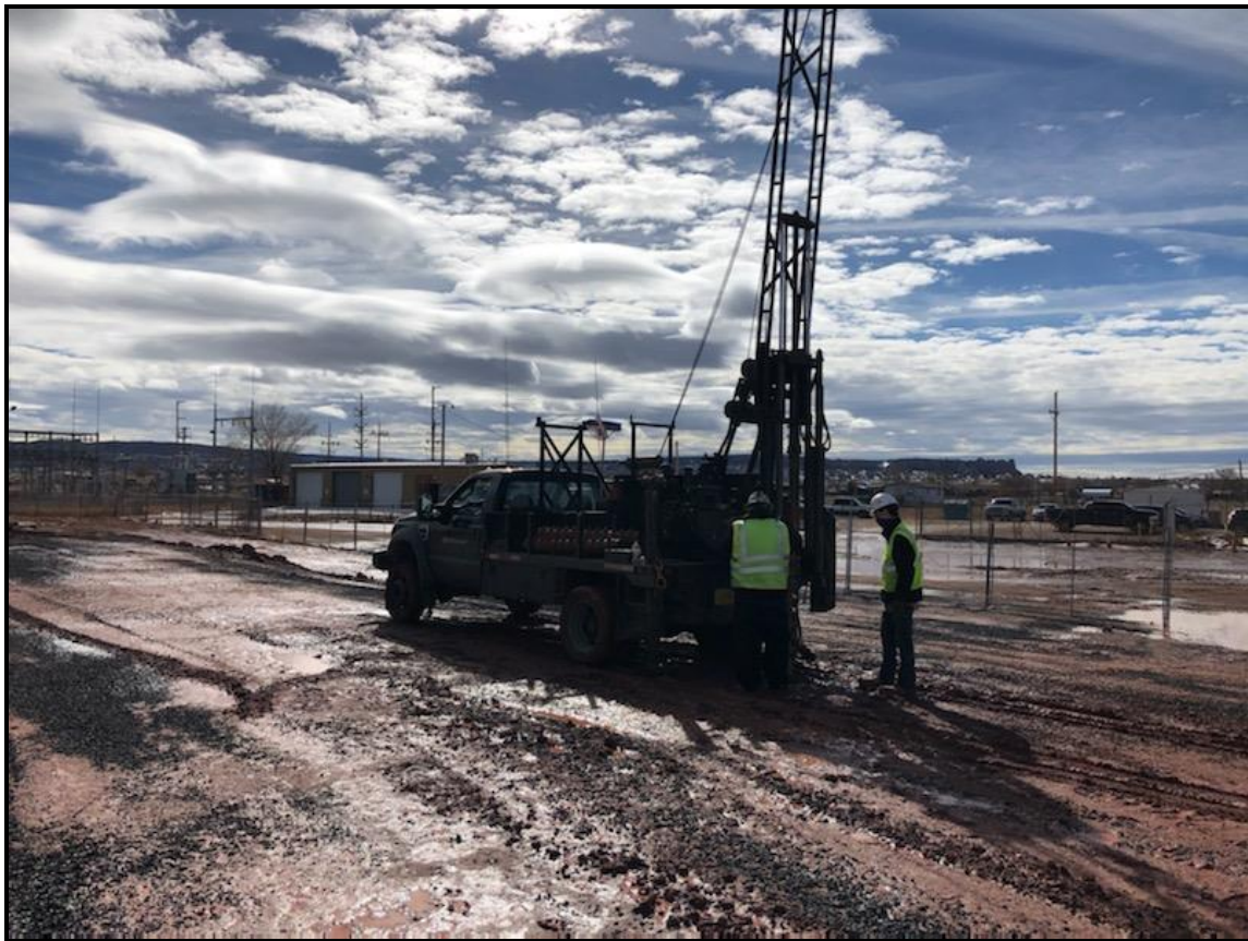
Drill Rig at Boring B-7 View to the Southeast
