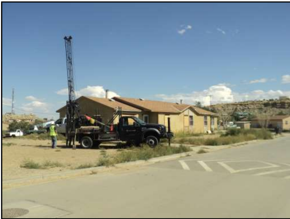
Drill Rig at B-4 View to the Southeast
