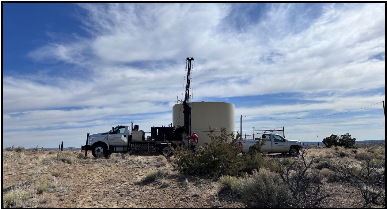
Drill Rig at Boring B-2 View Towards the East
