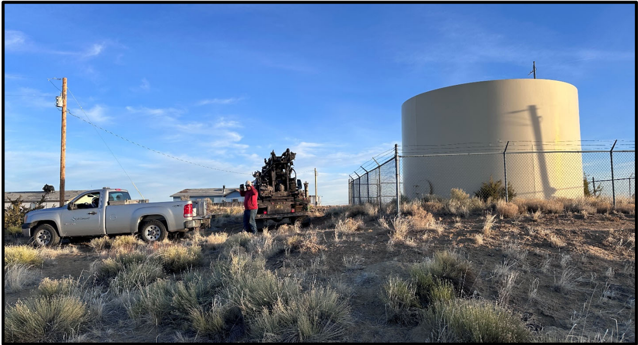
Drill Rig at Boring B-1 View Towards the North
