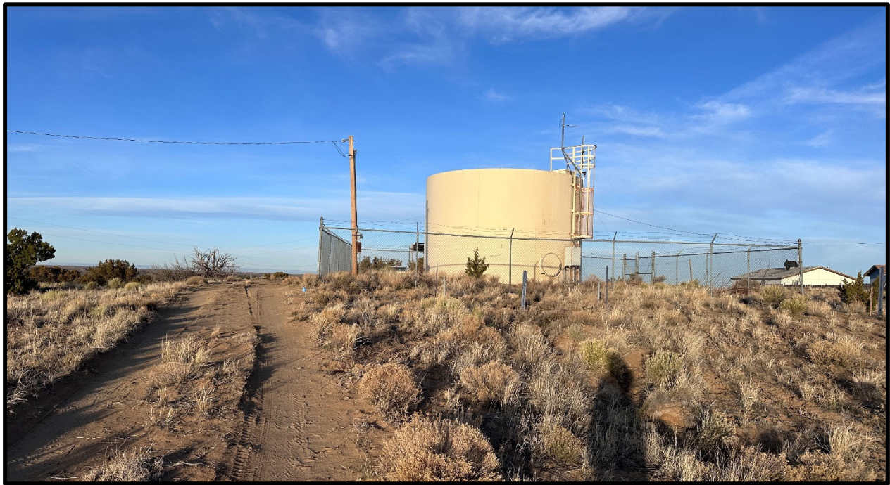
Existing Tank View Towards the West
