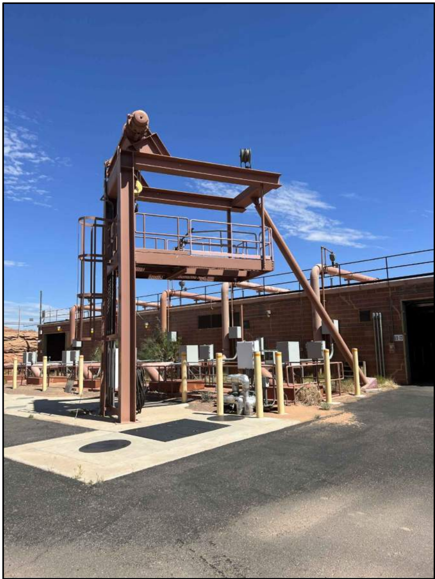
MOVEABLE FRAME & HOIST FOR PUMP EXTRACTION
