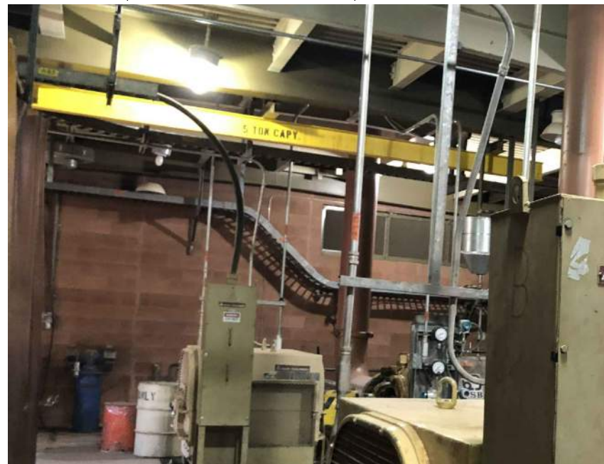
EXISTING 5 TON CRANE HOIST BEAM
