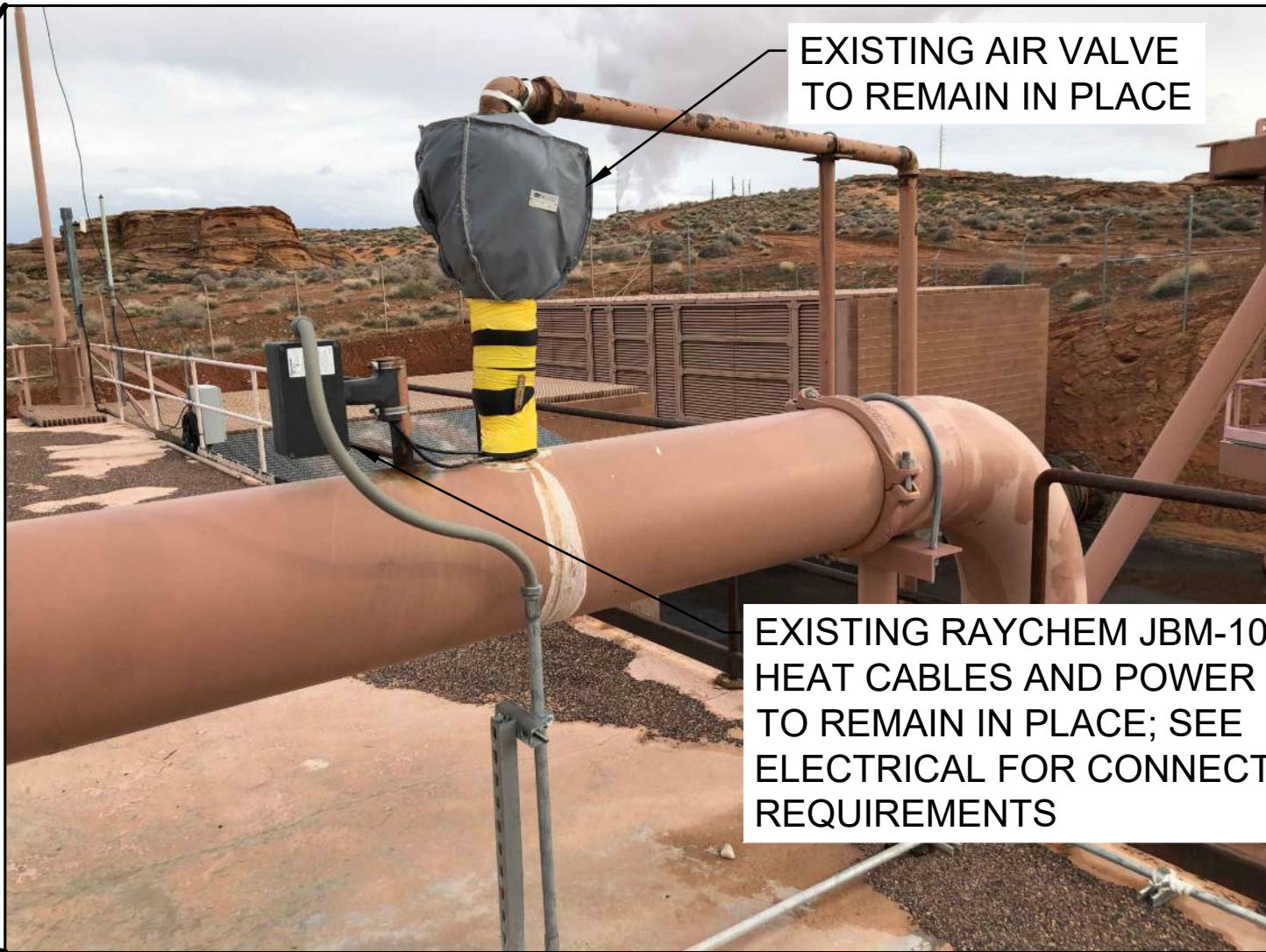
EXISTING SUBMERSIBLE PUMP DISCHARGE PIPE ON ROOF
