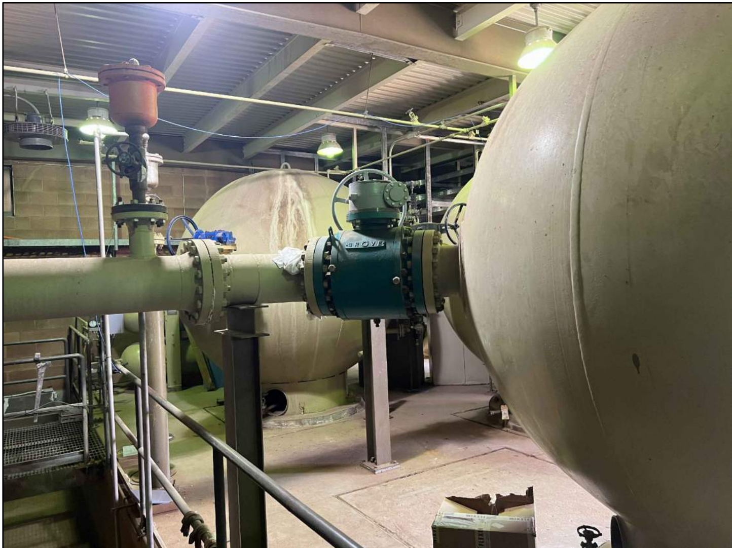
GENERAL DEPICTION OF EXISTING SURGE VESSEL AND PIPING
