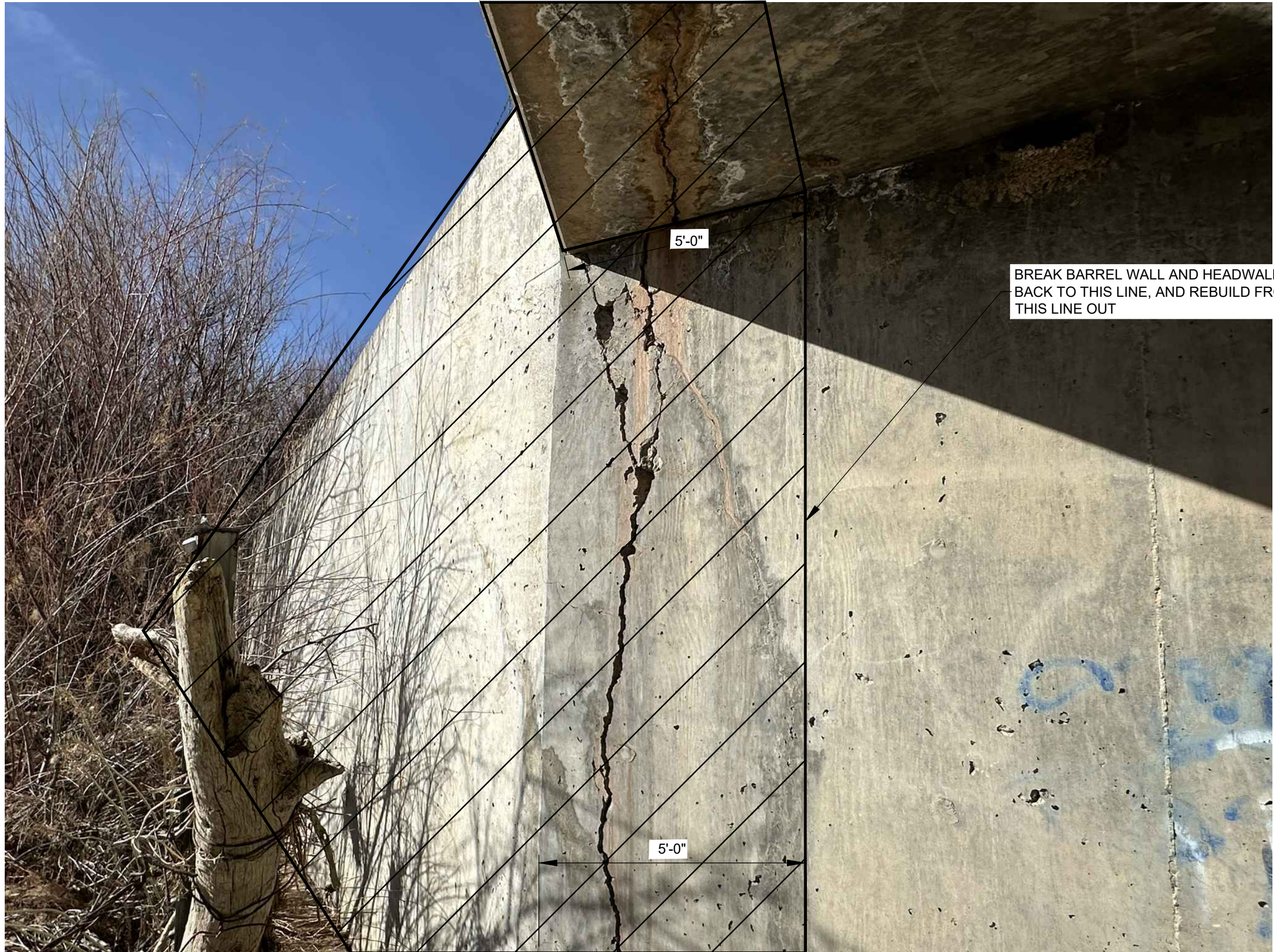
LIMITS OF WING AND BARREL WALL REMOVAL
