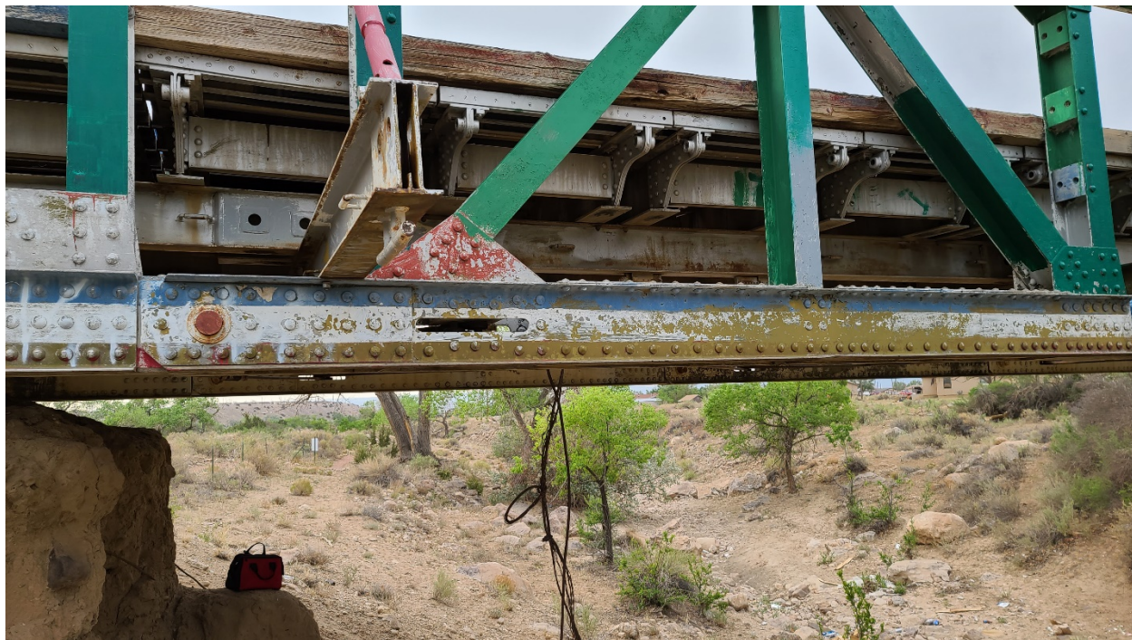
West Rail deck support system
