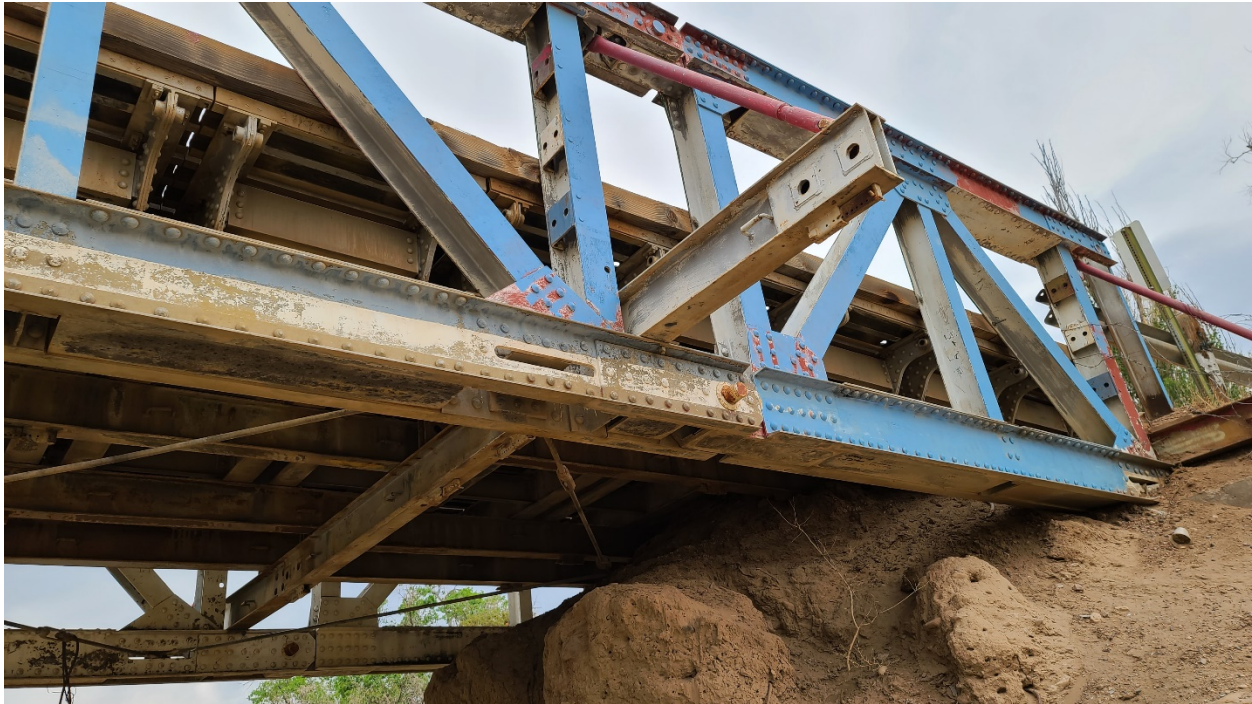
NE corner of bridge
