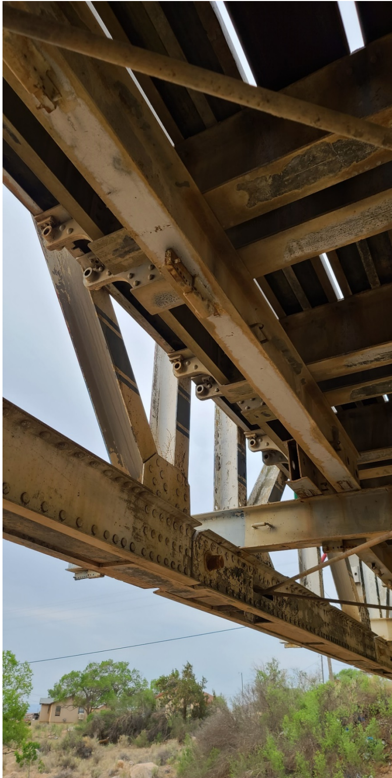
East Rail support structure
