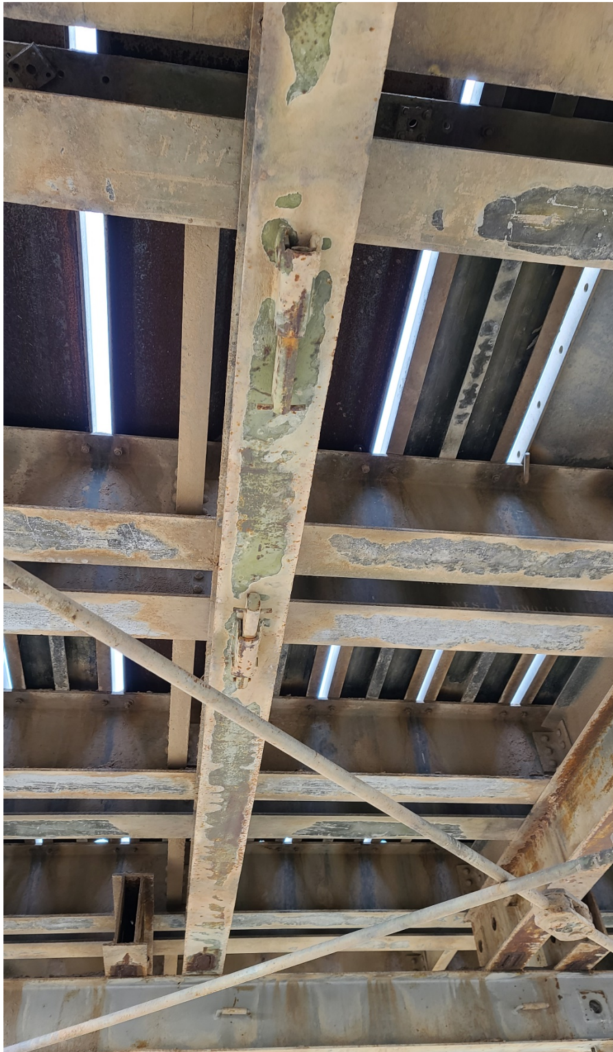
Underside of bridge superstructure
