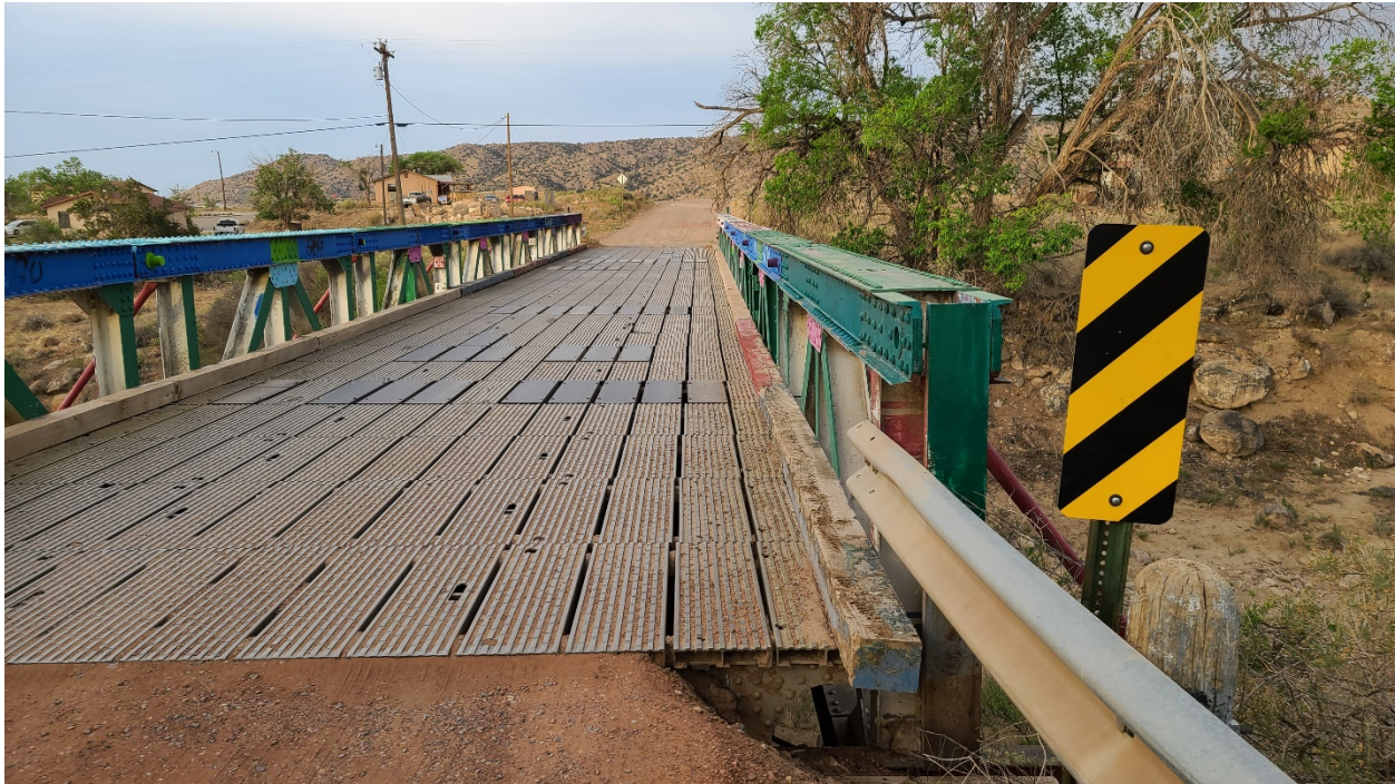
South end of bridge
