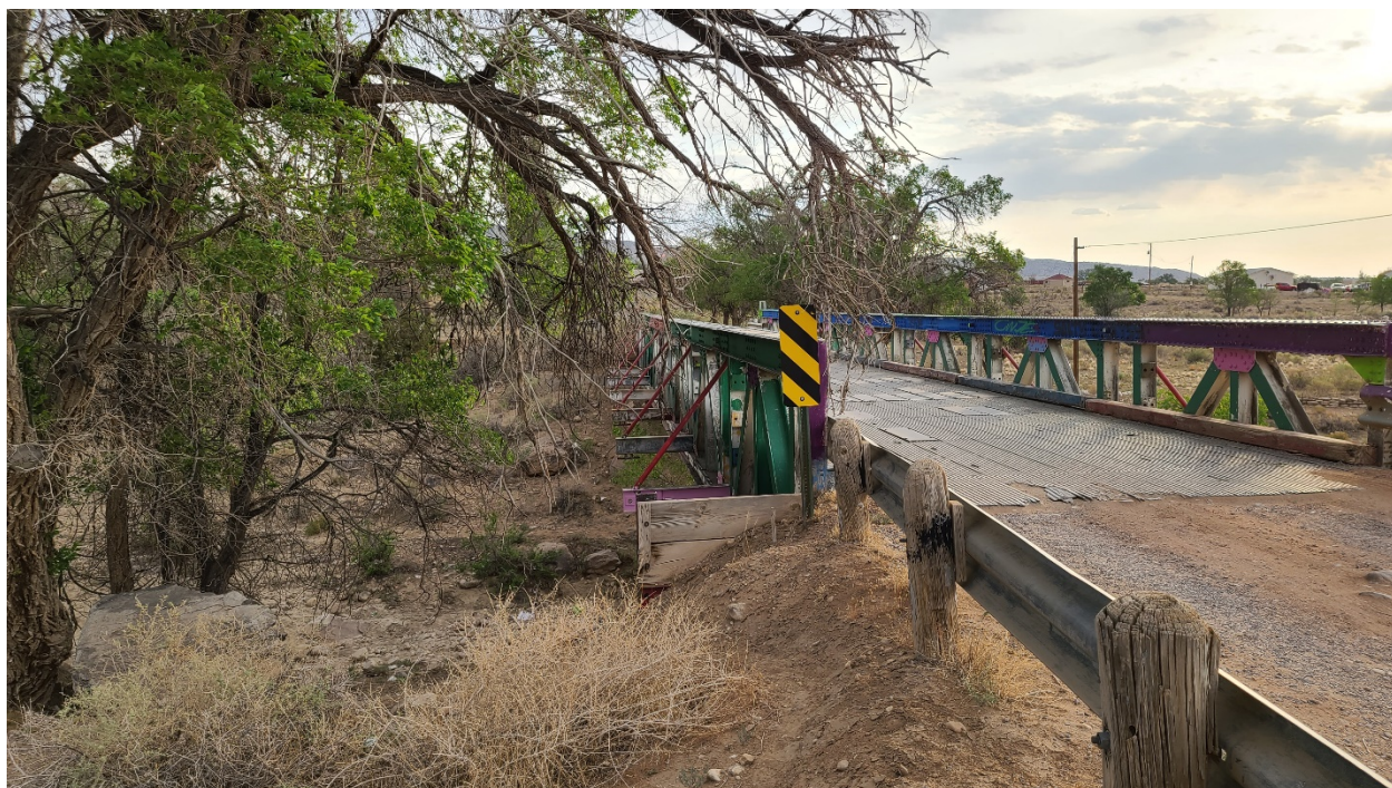
West Rail outside looking from South to North.
