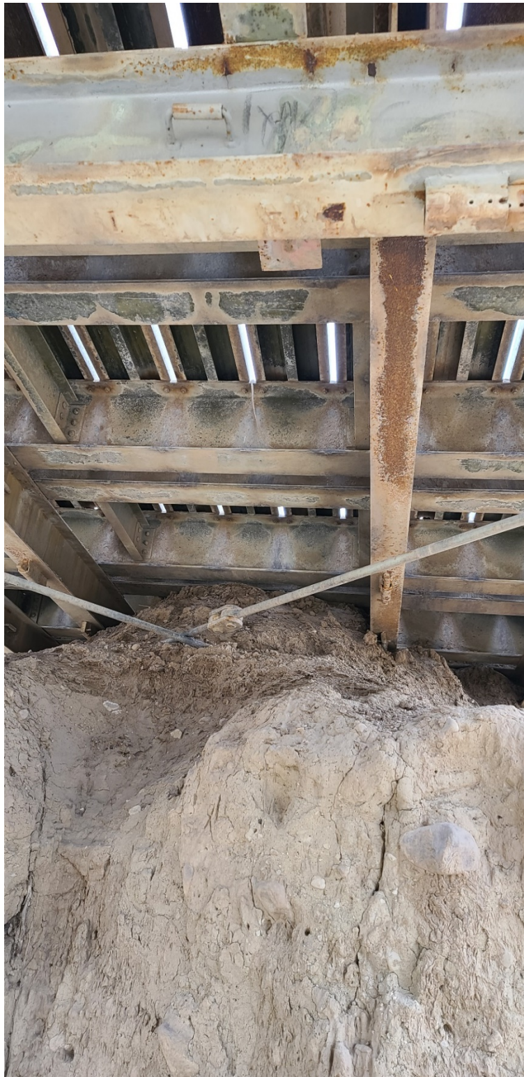
Underside of north end of bridge
