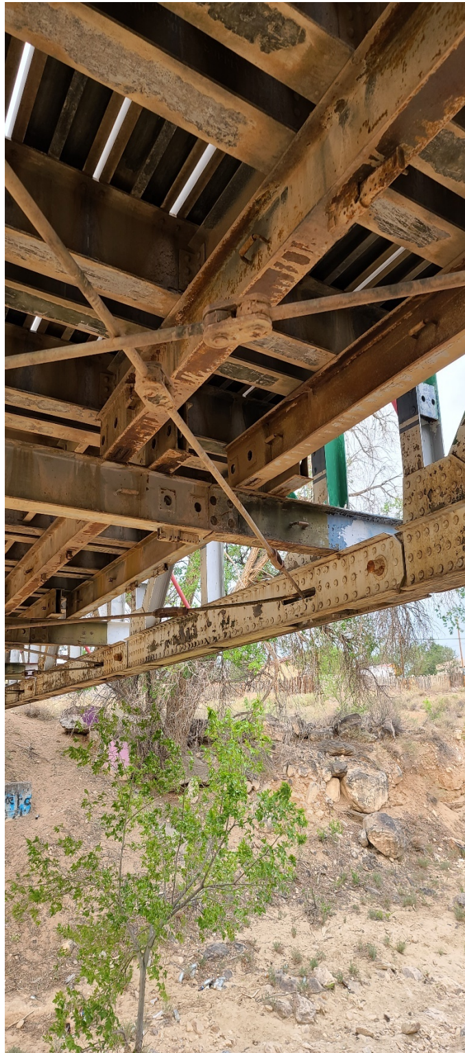
West Rail support structure
