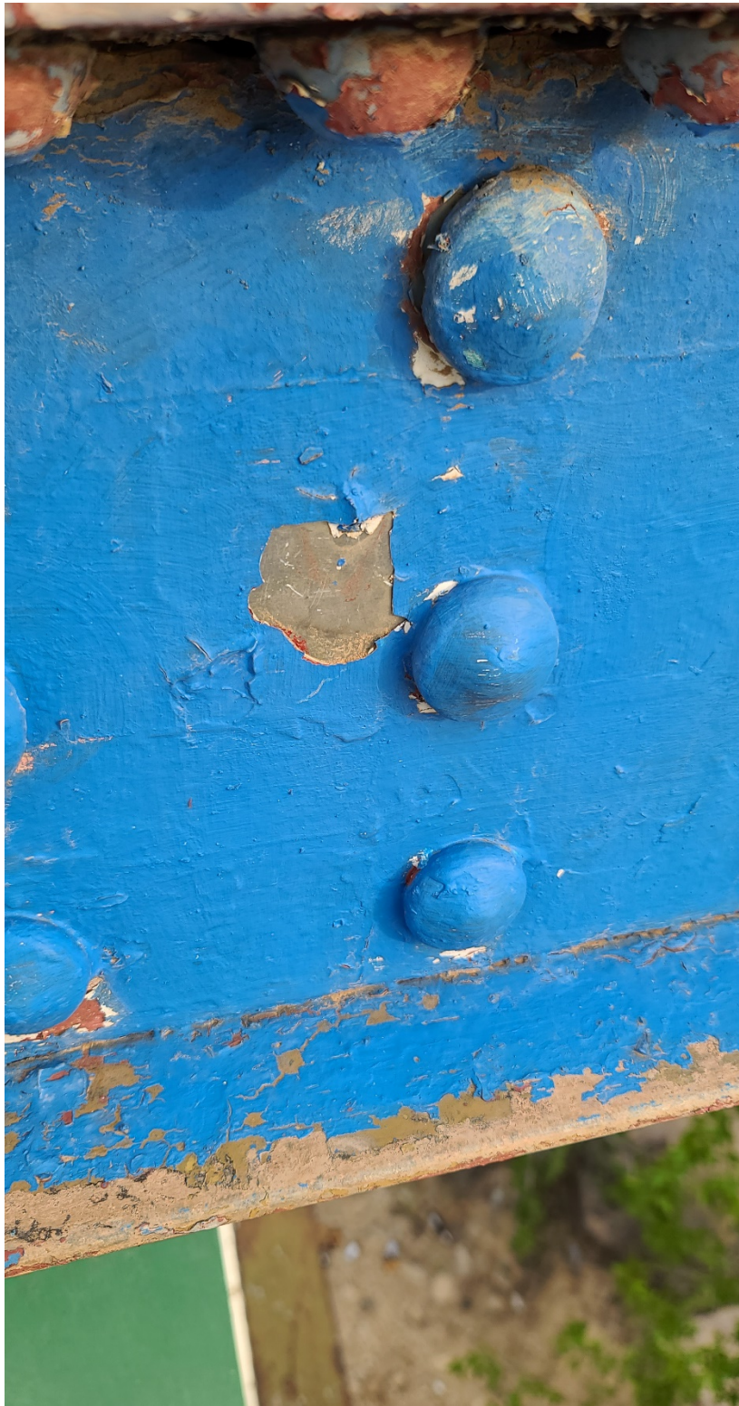
West Rail blue paint at mid span
