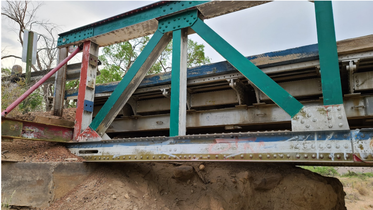
NW corner of bridge
