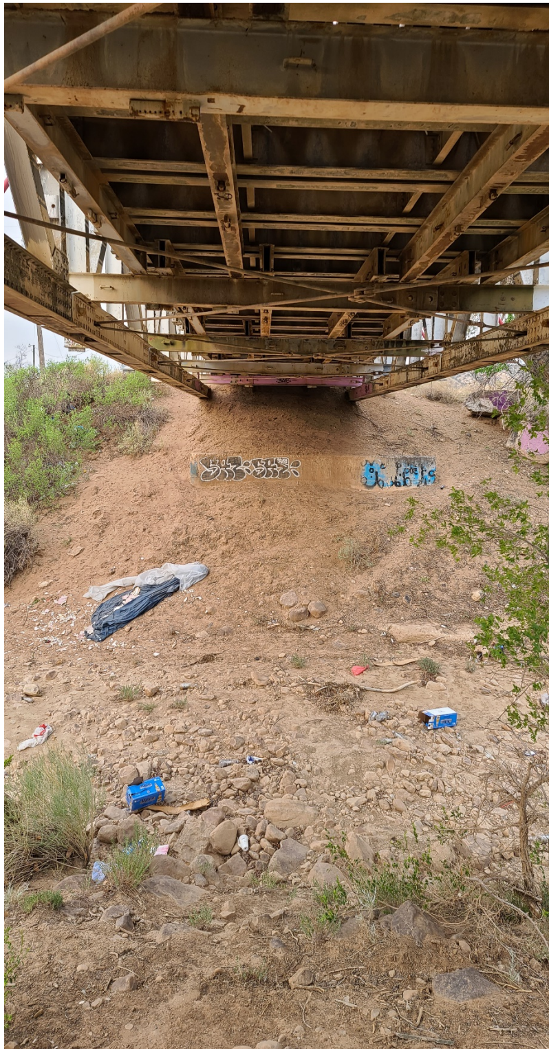
Underside of bridge from north looking south.
