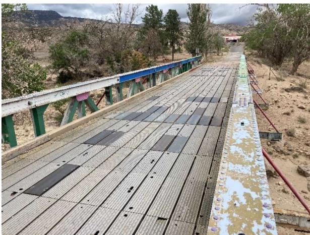
Photo 3. Looking north toward bridge with steel deck and guard rails.
