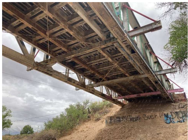
Photo 4. Photo of I-beams beneath bridge. Facing southwest.
