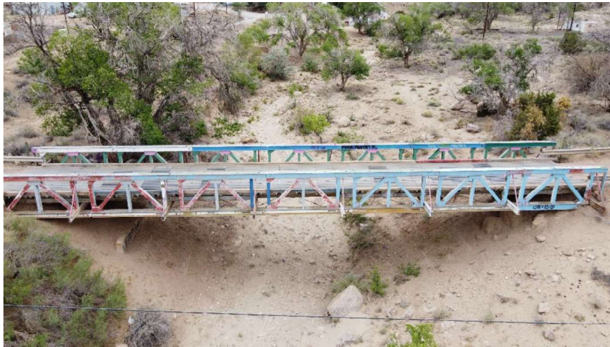
Photo 2. Overview of bridge facing west.
