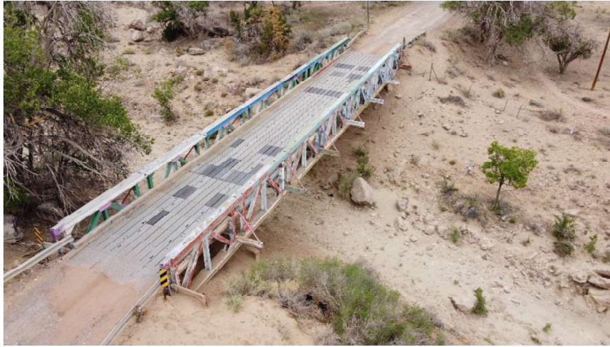
Photo 1. Overview of bridge facing north.
